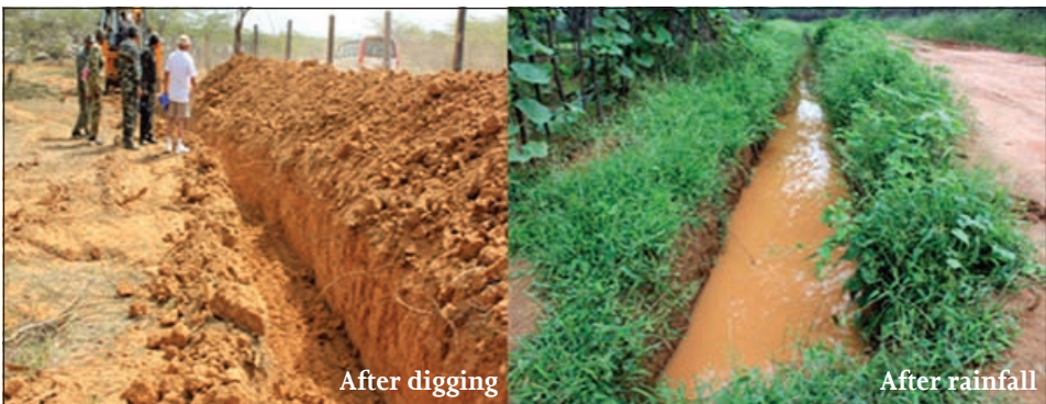
Figure 8: 10 km long trenching done to check rainwater runoff.
